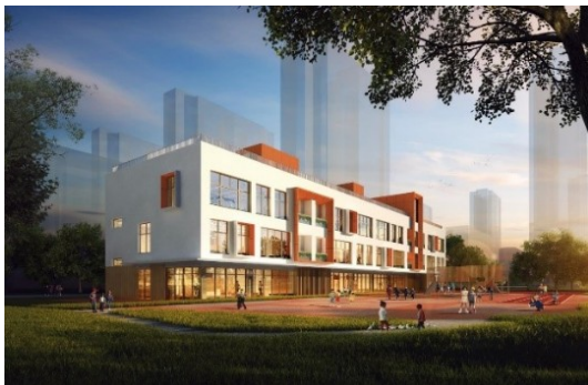
Kindergarten of Longfor Gaobeidian Railway City (China)
