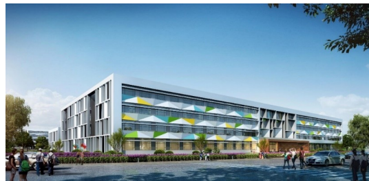
Primary School & Middle School in Sino-Singapore (China)
