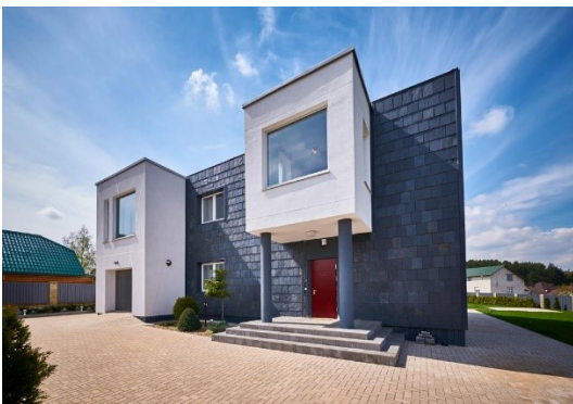
C2A Renovation (Belarus)
